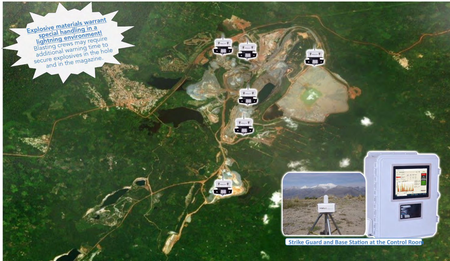
Figure 10: Lightning Warning System at Damang Mine
