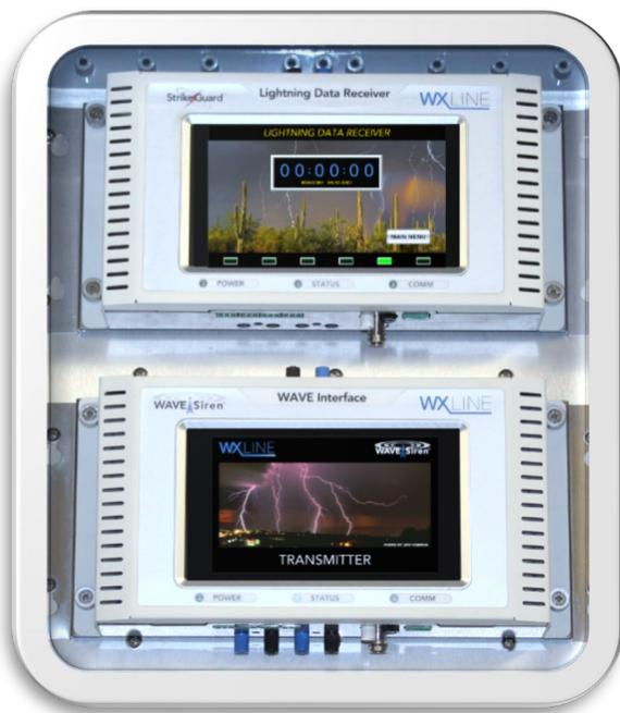
The Interface is normally mounted on a wall in an office environment and is often co-located with lightning detection equipment, with cable connections between the two pieces of equipment. It is important to bond the WAVE Interface chassis to the chassis of the Strike Guard Lightning Data Receiver to minimize the potential difference between these enclosures in the event of close lightning. At a minimum, a cable serving as a ground strap ties the two chassis together, electrically.
